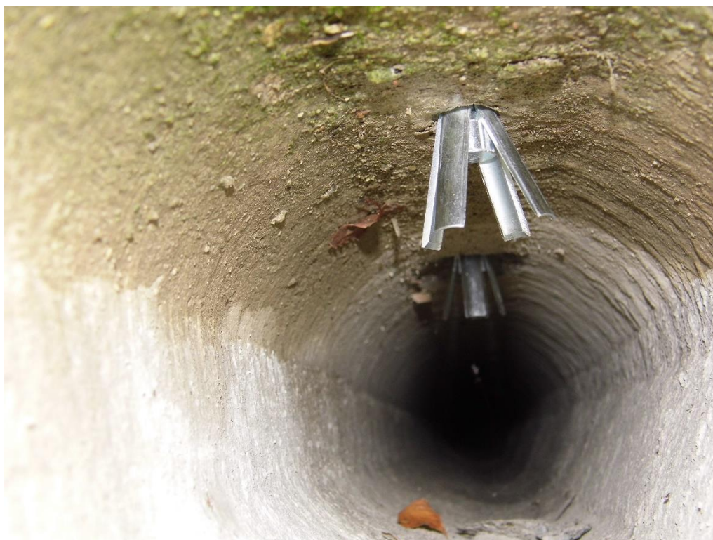
Figure 3. View of the anchor sleeve once fully tightened
